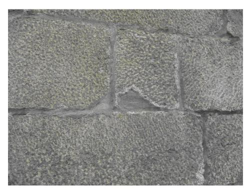
Figure 4.2.2.1 Connection between granite and mortar of the ruins of the St. Paul
