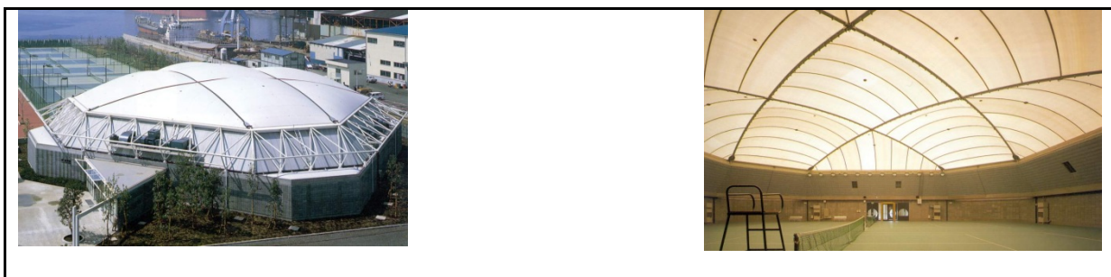
Figure 3-2: Pneus Single-layer pneumatic structure from the outside (left) and the inside (right)
