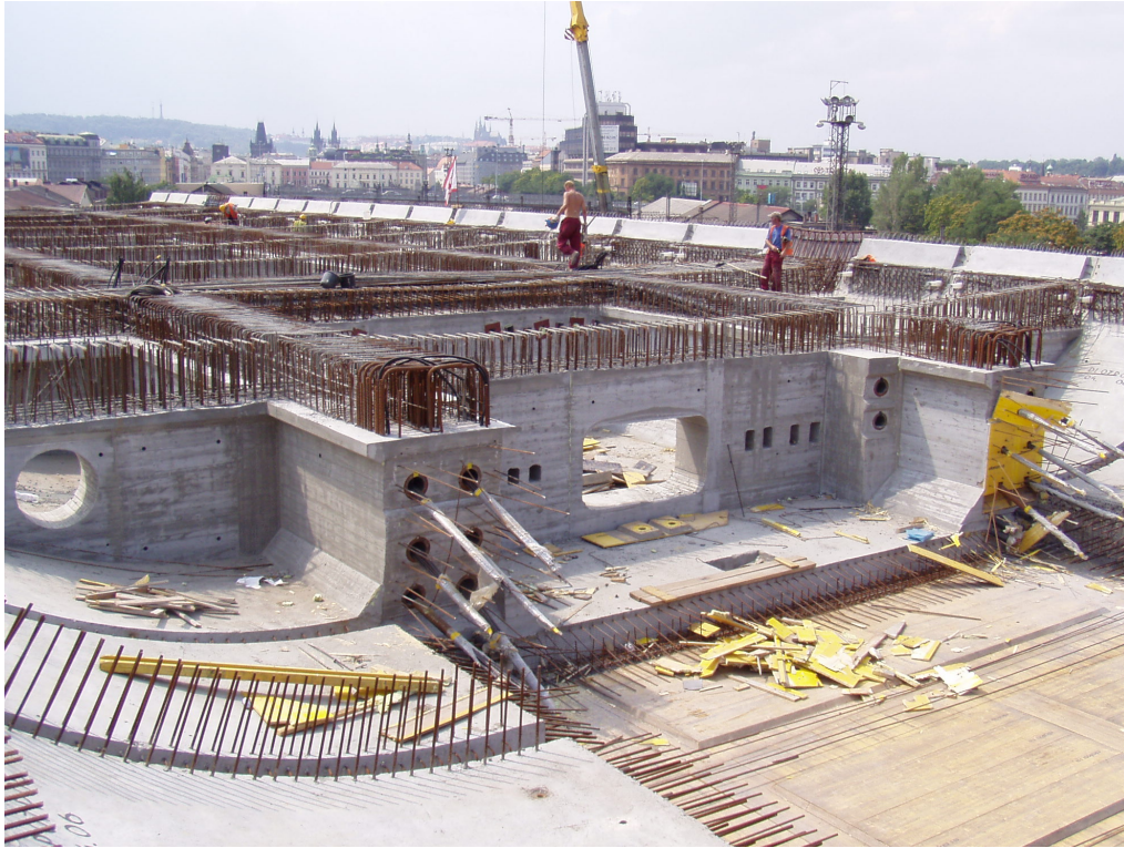
Figure 10: Construction of railway scaffold bridge (photo D. Prause)
