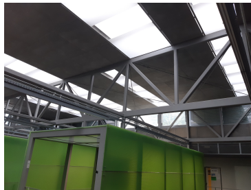
Truss structure in the atelier at Faculty of Civil Engineering
