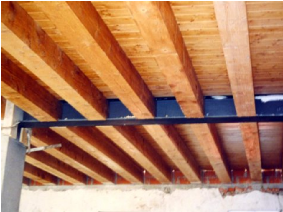
Figure 2.1: Timber and concrete composite schemes also enable large open-plan buildings to be constructed primary beams are then made of steel or glulam timber with a large cross-section
