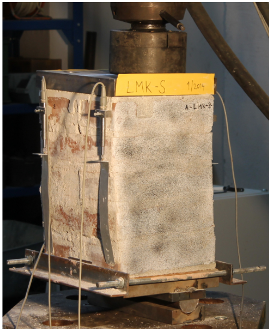
Figure 5.4: Tested masonry pier subjected to the combination of compression and bending, introduced via eccentric loading and supporting.
