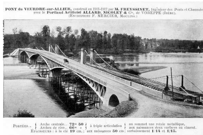
Figure 1.1: Veudre bridge over Allier (1911–1912) designed by E. Freyssinet [1], flattened three-span arch concrete bridge with central span 72.5 m; increasing deflections caused by shrinkage and creep (12 - 13 cm in three years); problem solved by additional thrust jacks in the center of the arches.
