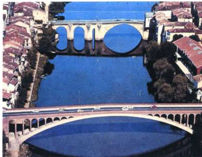
Figure 1.2: Bridge at Villeneuve-sur-Lot (1914–1920) designed by E. Freyssinet [1], plain concrete arch bridge with 96m span; decentering jacks at the crown introduced already in the design phase.
