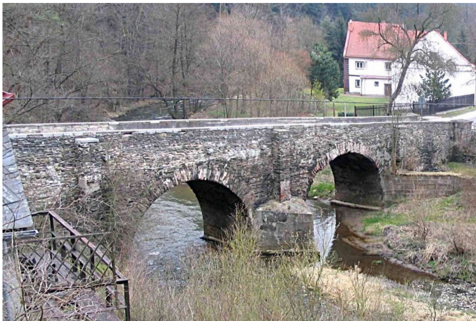
Figure 5: Rabštejn bridge. Recent photo (Pudis a.s., 2015)
