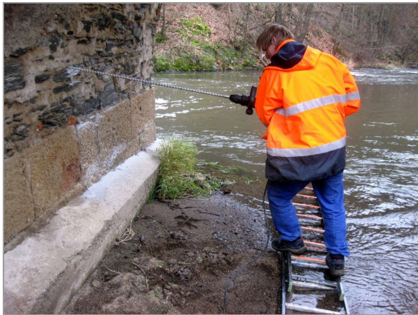
Figure 14: Diagonal drilling in central pier (Pudis report, 2015)
