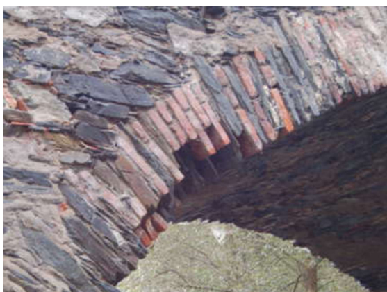
Figure 6: Brick portions in phyllite masonry arch (Pudis a.s., 2015)
