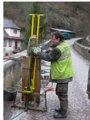
Figure 12: Drilling equipment (Pudis a.s., 2015)
