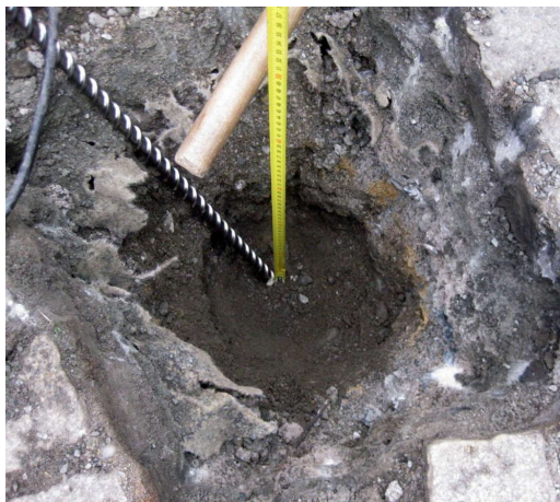
Figure 11: Roadway pit (Pudis a.s., 2015)
