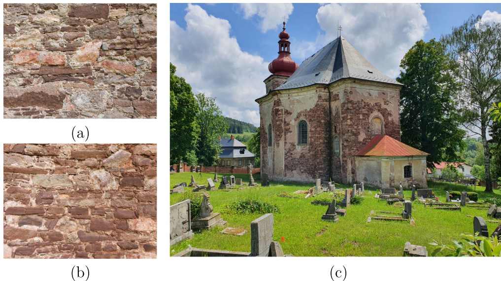
Fig. 2. (a)-(b) Examples of irregular masonry panels, (d) Church of All Saints, Heřmánkovice, Broumov.
