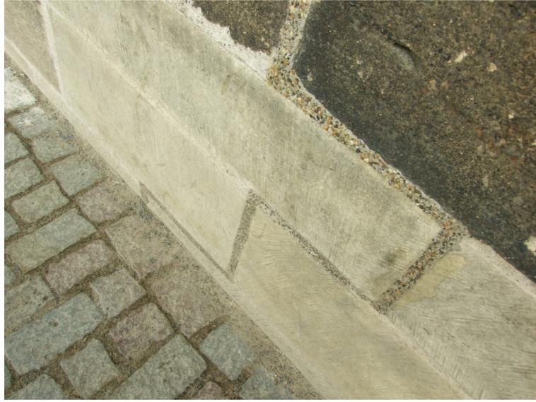
Figure 5: Dilatation joint and contrast between old and new blocks [5].
