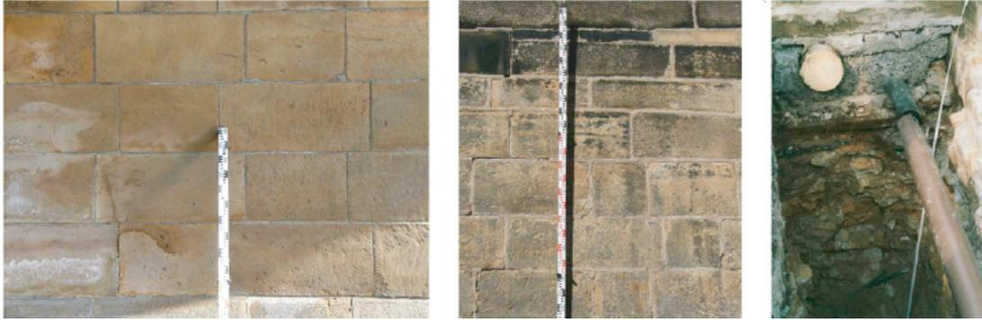
Figure 3: Periodic sandstone, non-periodic sandstone and filling masonry in the Charles bridge [5].
