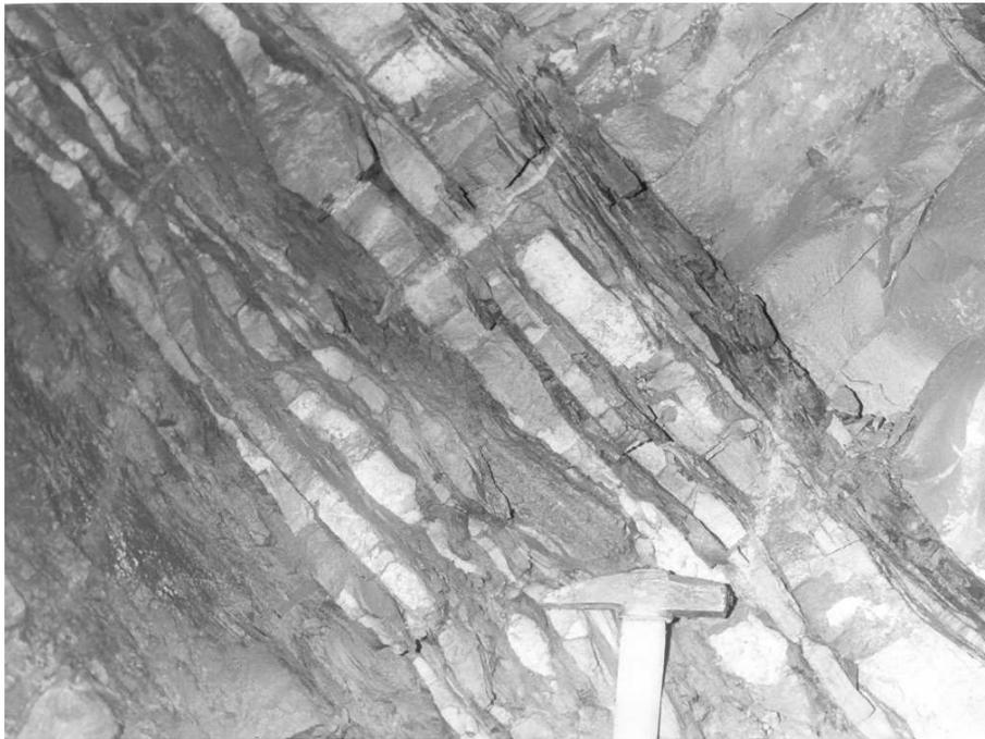
Figure 4.3: Detailed character of the Letná flysch strata with alternating schist and quartzite strata in the section under Pier No. 4.
