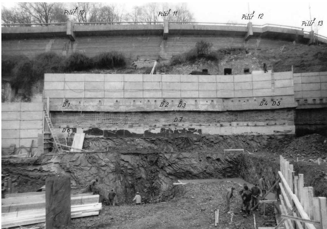
Figure 4.2: View of the excavation and temporary retaining structures of the hotel site. The elevated road is at the top.
