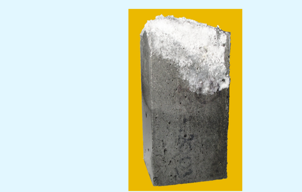
Typical efflorescence in a moisture-gradient environment.
