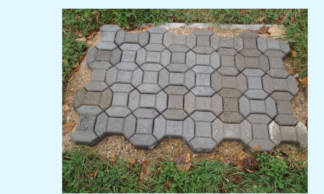
Pavement prototype after 22 weeks of exposure to weathering conditions.
