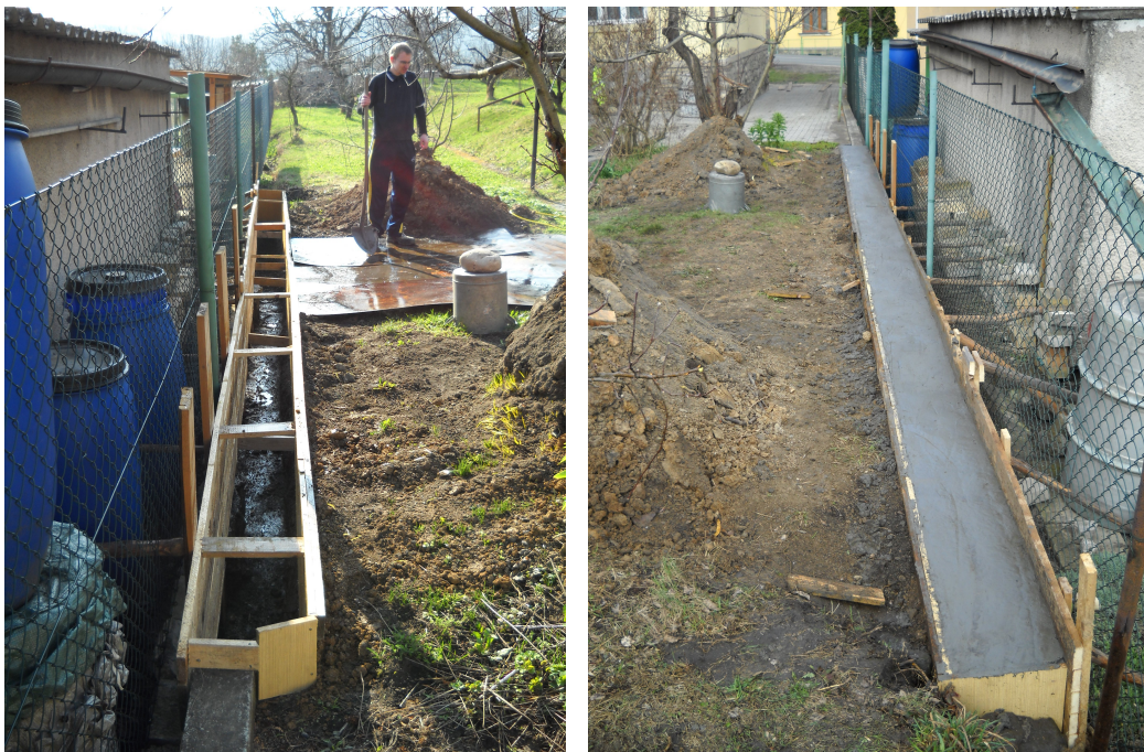
Figure 21: Wall before and after AAFA casting.
