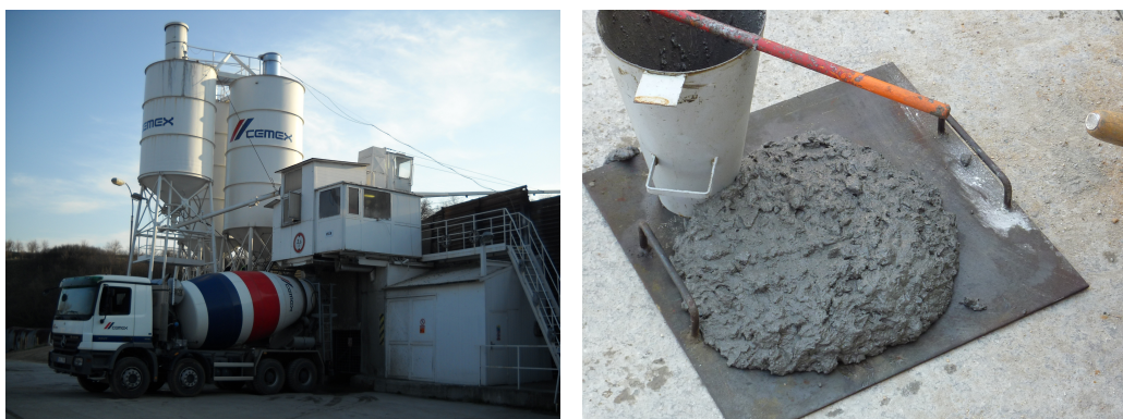
Figure 19: Left concreting plant, right flow test. Three cubic meters of AAFA concrete were produced, the volume of blender in the concreting plant is 0.33 m 3 , eight mixtures had been done to fill the concrete agitator. The time elapsed between first and last mixture was approximately one hour.
