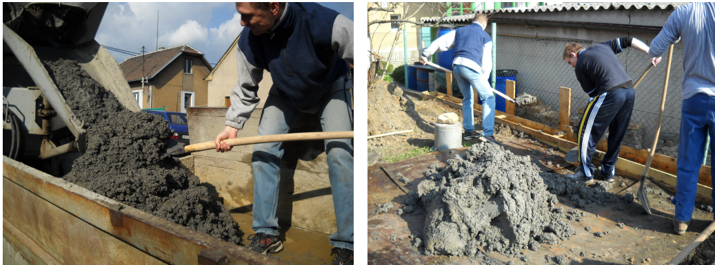
Figure 20: The workability of AAFA concrete was not ideal one hour after mixing.
